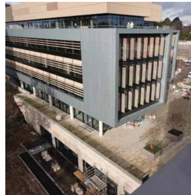
A bird's eye view of the almost finished Southampton GTC
